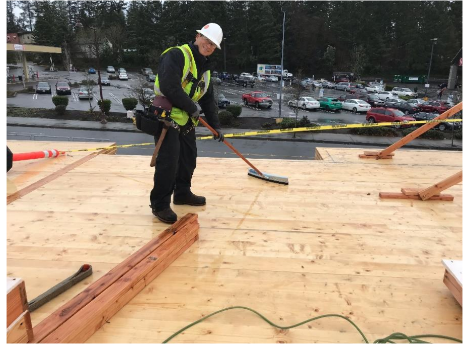
Photo 4: Squeegee use on wet CLT panel.
