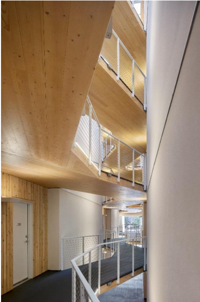
Photo 1: Example of exposed CLT installation at finished project. The Canyons, Portland, Oregon.
