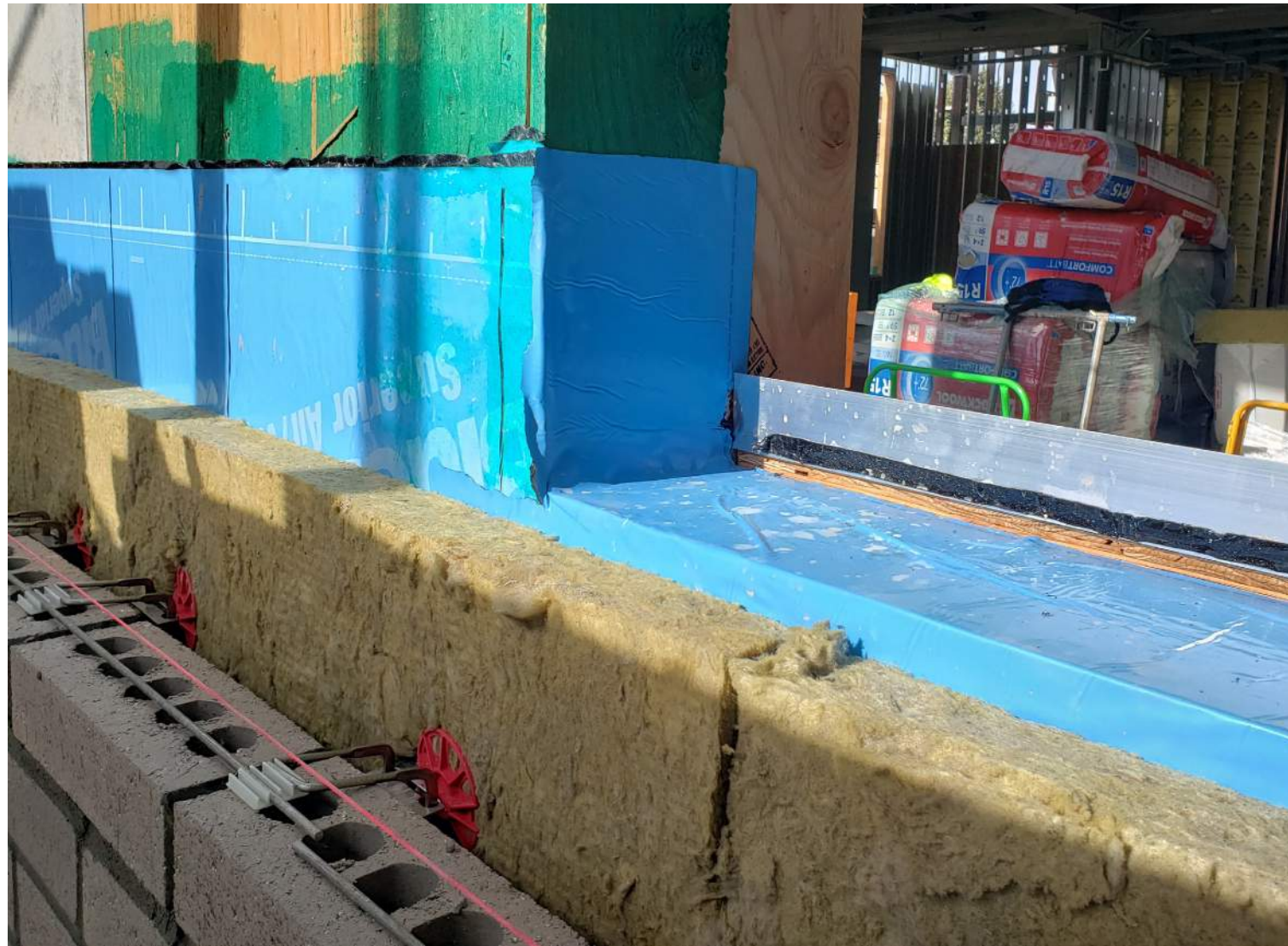
TYPICAL EXTERIOR PASSIVE HOUSE WALL (R-46.6)
