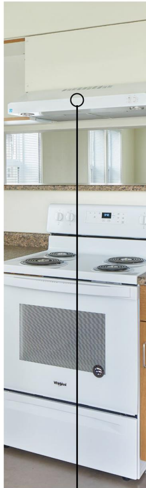
Bathrooms fans and kitchen hood fans are routed directly to the exterior
